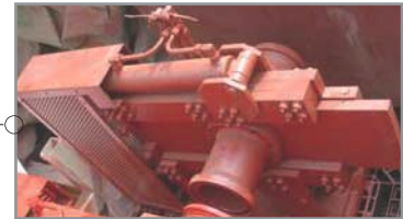
HYDRORIC SHUT OFF VALVE AND DIVERSION VALVE
